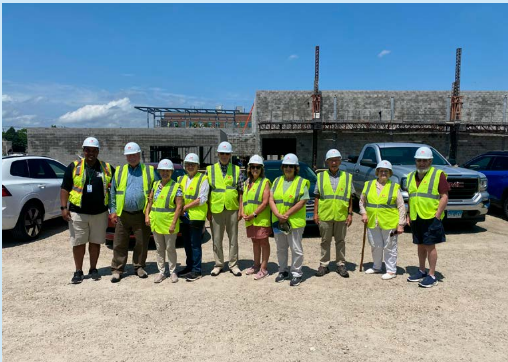
In the absence of our regularly scheduled meeting, New London Rotarians got a sneak-peek at the New London Community Center construction site last week. Thanks to those who attended and to the City for offering the tour. Visit the Club's Facebook page for additional photos.
