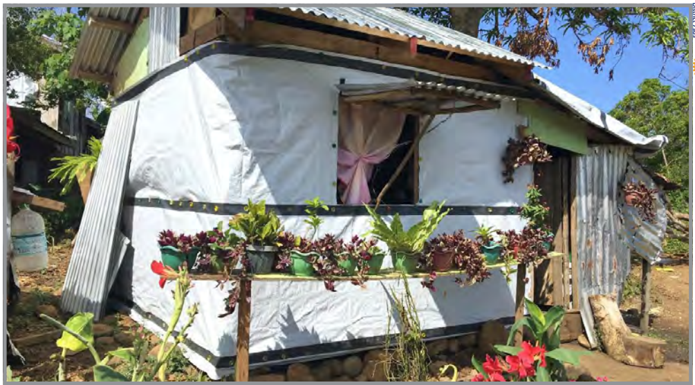
A family home in the Philippines, built by a mix of local materials and the tarpaulins from a ShelterBox kit. This family certainly takes pride in their new makeshift home, built after they lost their own in a recent storm. Article by Michele Papakie
