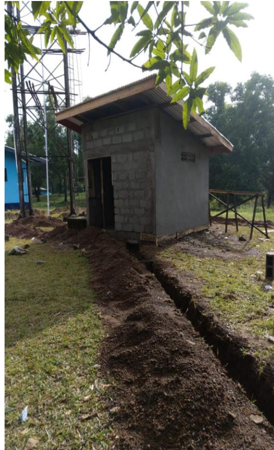
A new deep well is being dug. During the rainy season, the shallow wells would become contaminated. Trenches are dug for piping.
