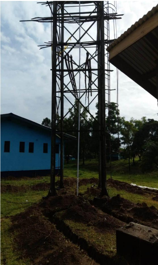
A new deep well is being dug. During the rainy season, the shallow wells would become contaminated. Trenches are dug for piping.
