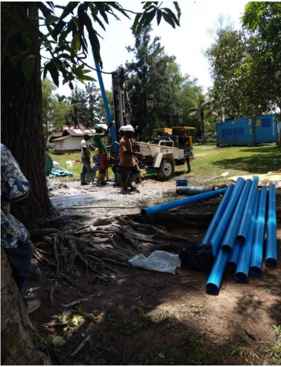
A new deep well is being dug. During the rainy season, the shallow wells would become contaminated. Trenches are dug for piping.
