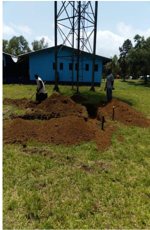
A new deep well is being dug. During the rainy season, the shallow wells would become contaminated. Trenches are dug for piping.
