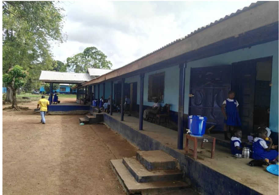
the school without running water, pipes were broken
