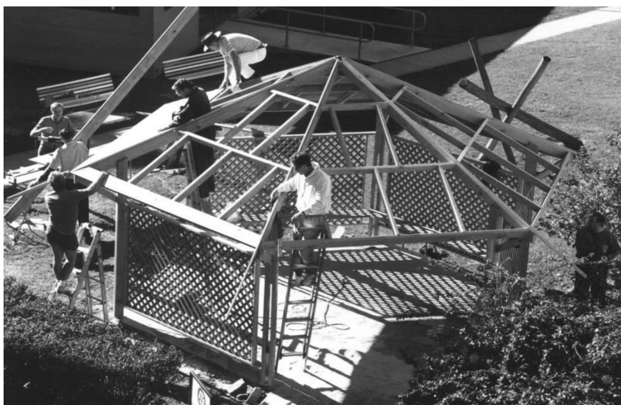
The Rotunda at Nepean Hospital under construction.
