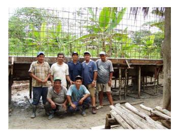
Construction continues on the water tank at Nuevo Progreso, Peru. Here is the construction crew in front of the water tank. APECA Projects Coordinator Pablo is in the back row second from right. Note the extensive rebar cage to support the cement walls of the tank.
